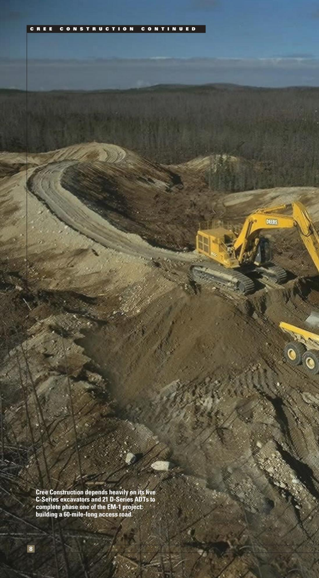
Cree Construction is deploying a battalion of Deere equipment to complete the project, including five C-Series Excavators, 21 D-Series Articulated Dump Trucks (ADTs), one 544H Wheel Loader, one C-Series Dozer, and three 772CH Graders.
